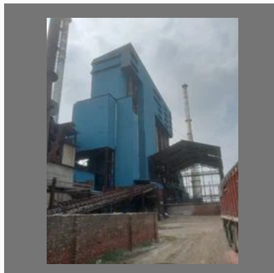
Sheet Metal Roofing Fabrication Work
