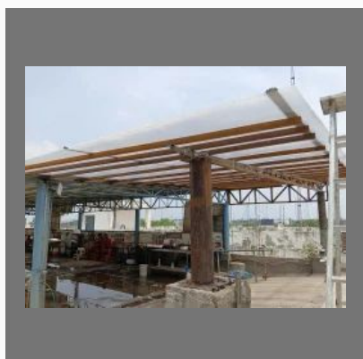
Mild Steel Shed With Multiwall Sheet
