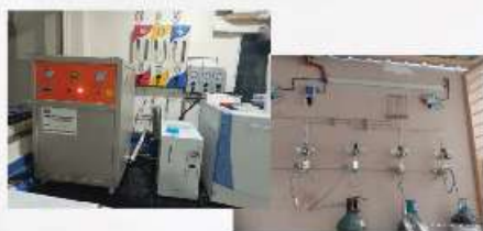
Gas Line Installation
